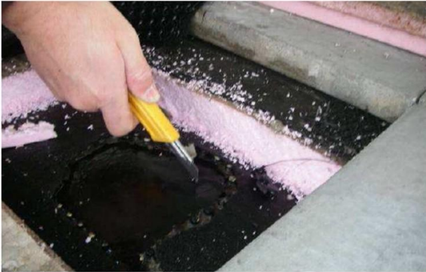
Figure 11 & Figure 12: Cutting of Membrane Blister and expulsion of water during extraction process.
